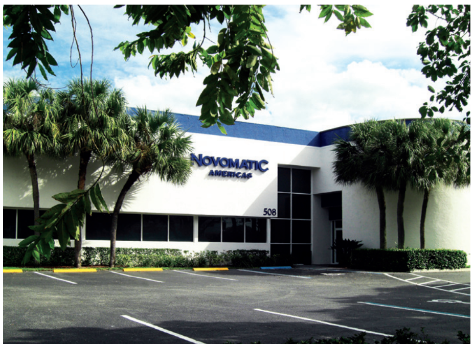
NOVOMATIC Americas headquarters in Deerfield Beach, Florida.
