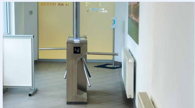
A turnstile in front of the staff restaurant temporarily blocks access when a critical threshold of 100 people is reached inside.
